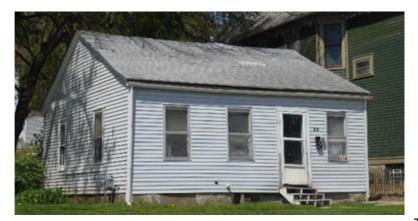
Figure 5. The Dietrich Tegrunde House, 1863. Increasingly rare antebellum example of workman's house in the district. Wood clapboard concealed by asphalt brick underneath aluminum siding. Functional rental at the time of demolition. Demolished 2015 to create green space.
