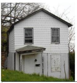
517 Ripley Street. 1850s-60s. Hamburg. Post and beam construction. Wood clapboard concealed under asbestos and rolled brick siding. Undergoing rehabilitation. Author Photo.
