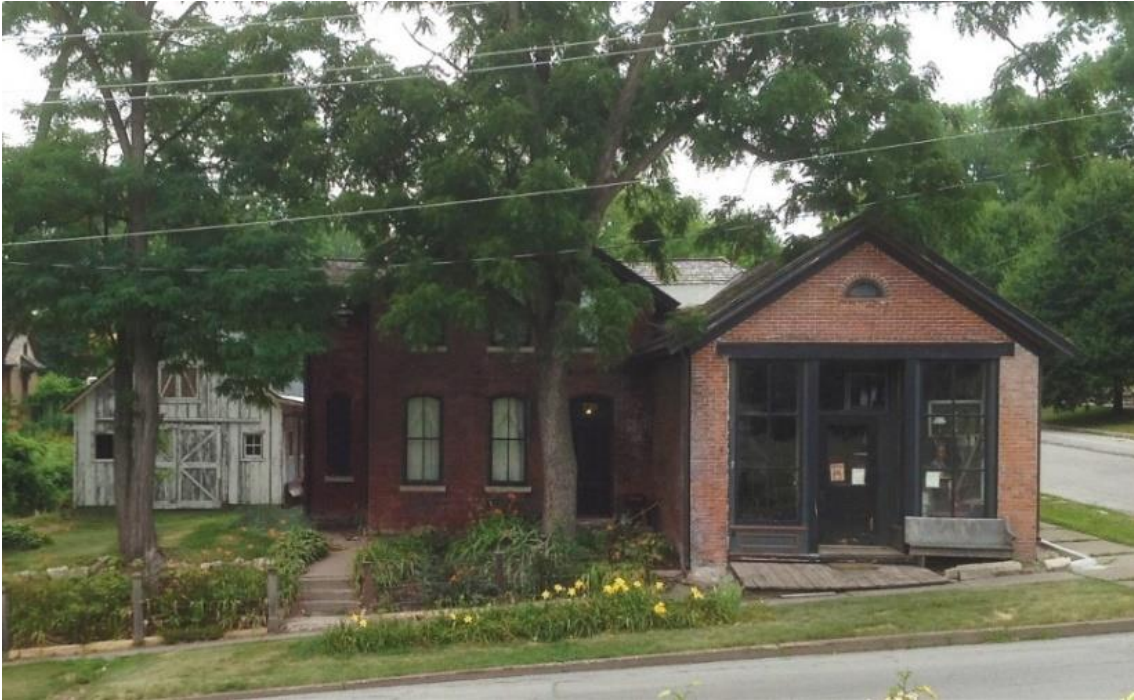
The Jipp Home and Grocery 732 Gaines Street
